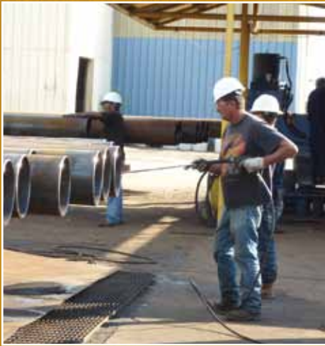
Lubricant is removed from the pipe after the "bell" end is formed.
